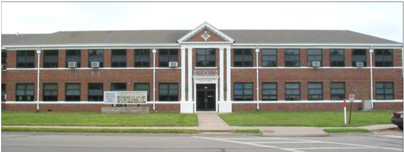
Andale Rural High School — photograph by Brenda Spencer of Preservation Planning and Design, taken May 10, 2004
